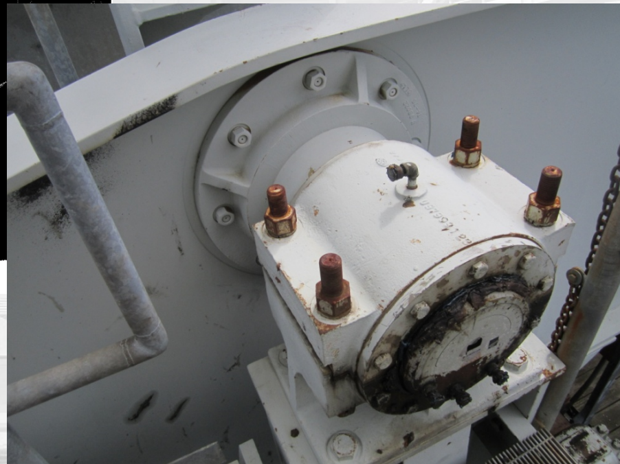
Figure 2.8.2.3.3-1 – A bascule bridge split sleeve type trunnion bearing
